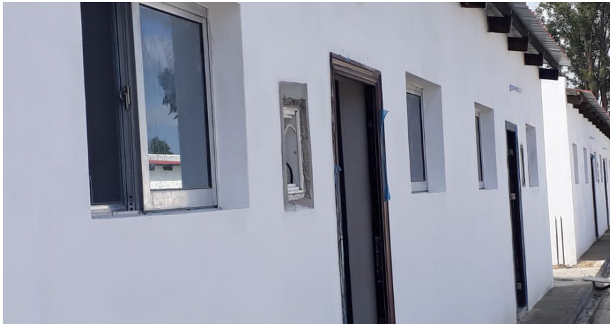
Image 1: Casa Real's homes ready for clients to move in.
